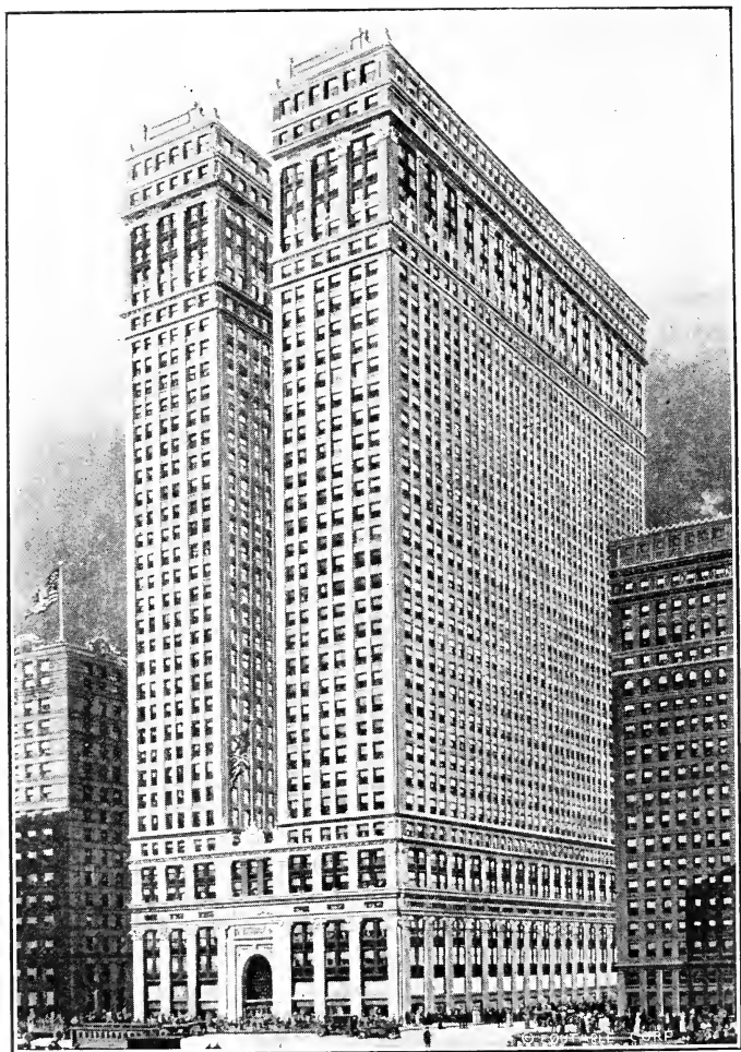
EQUITABLE BUILDING, Broadway to Nassau St., Pine to Cedar St.
